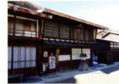
4 Nakamuras' Residence (Shioiri City) D-3 Typical machiya-style home from the Edo Period that belonged to a comb wholesaler.
